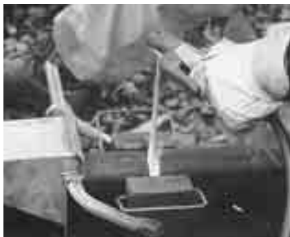
Joining of rails by mould welding: OK 74.78.
