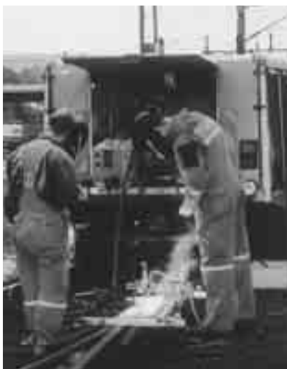
Mechanized welding: Railtrac BV/OK Tubrodur 15.43.
