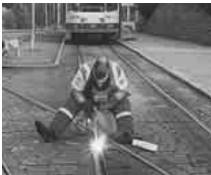
Tram line repair: OK 67.52.
